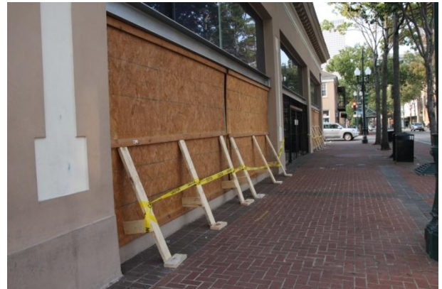
Figure 1. Boarded glass store front in Louisiana FEMA News Photo
